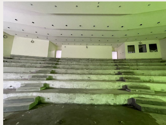
4/5F階梯教室地坪粉刷
